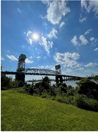
Figure 1: Cape Fear Memorial Bridge (view East-West)
